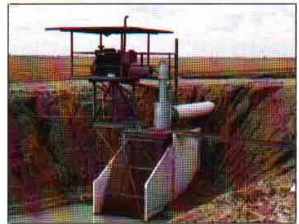
The model 21/24 cotton re-lift pump at Moree, NSW, Australia, has a diesel angle gear drive with below surface discharge, this system pumps 800 litres/second with 5 metres Total Dynamic Head.
