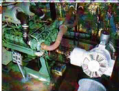
One of three model 21/24's pumping 1000 litres/sec with 16 metres Total Dynamic Head from the McIntyre River, Boggabilla, NSW, Australia. This river has a 12 metre water level variation.
