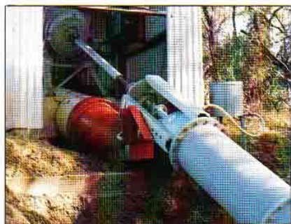
This 14/16 model, operating at Conargo NSW, Australia, has a direct coupled electric universal drive and pumps 450 litres/second with 7 metres Total Dynamic Head.
